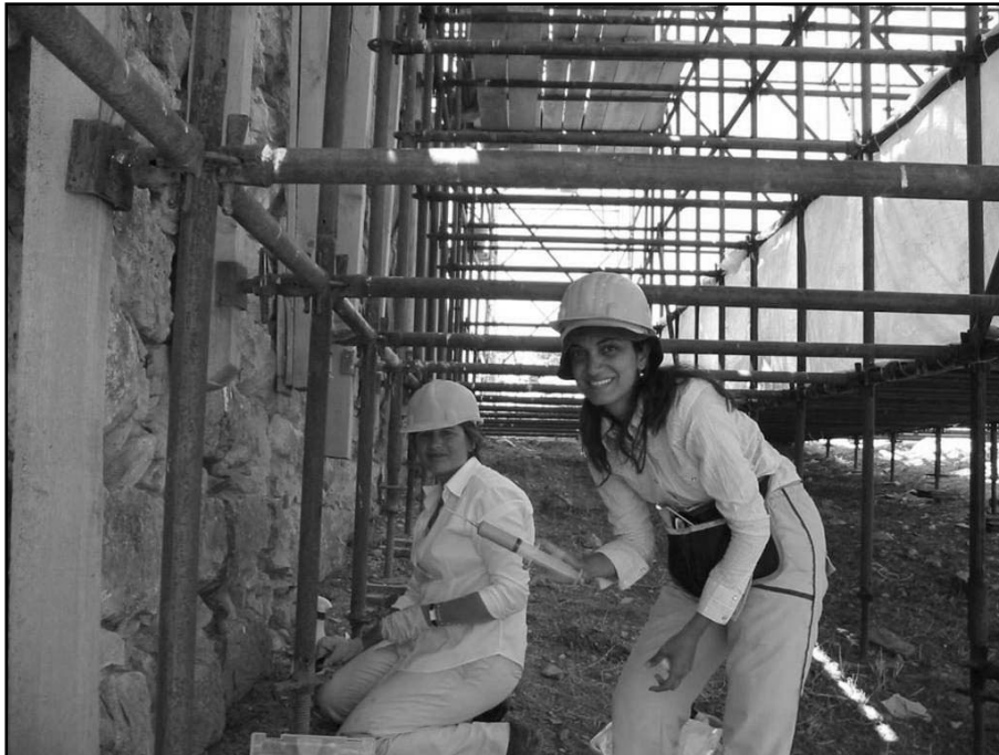
Fig. 13: Micro-grouting in the Citadel Gateway
