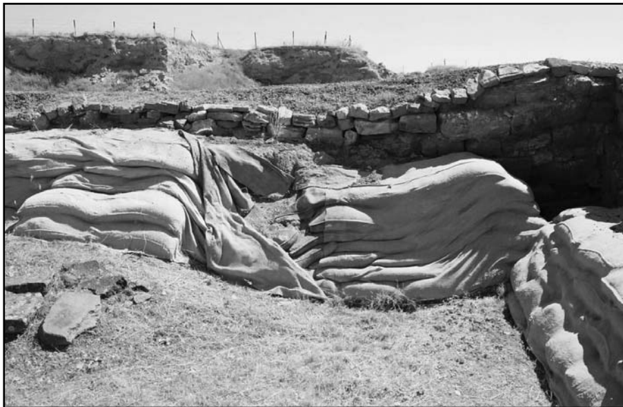
Fig. 14: Fate of sandbag buttresses in the Terrace Building
