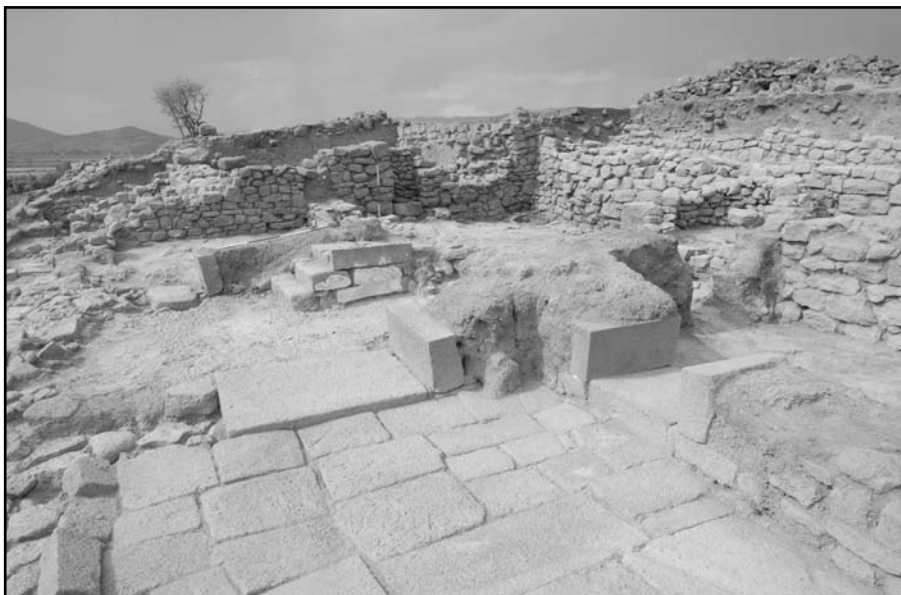
Fig. 6: The residency in area K-5 from northeast, MB II; in foreground stone-paved courtyard L.891, behind which rooms L.953 and L.1423 are visible; in right background wall W.1433 with its blocked doorway
